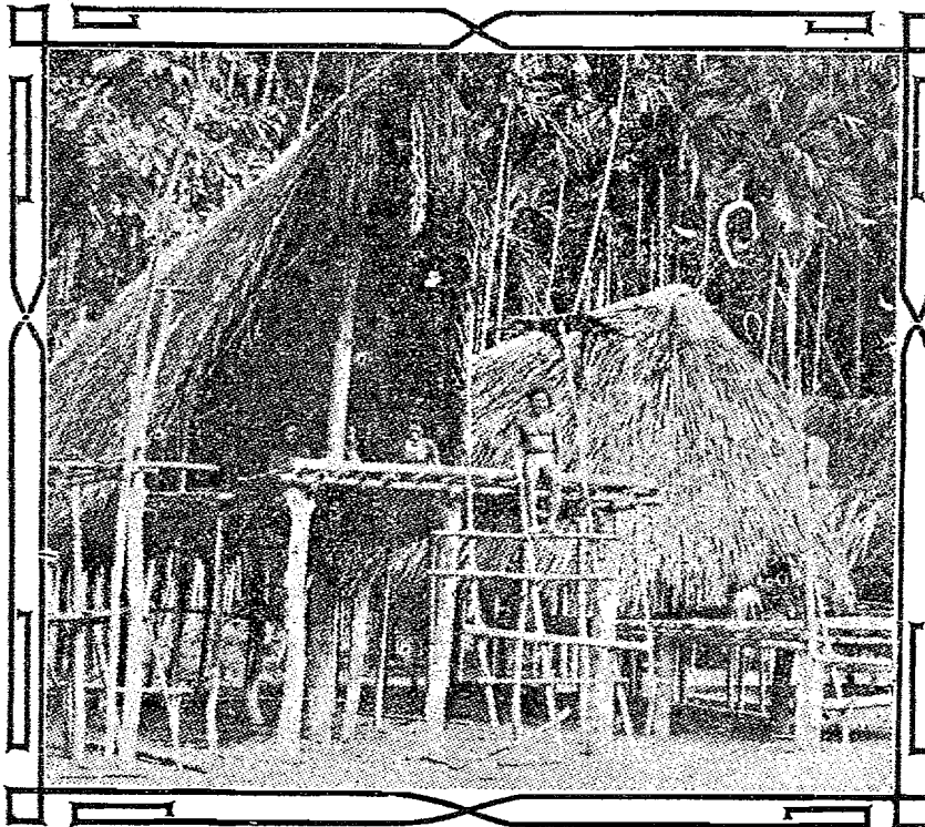
TYPICAL NEW GUINEA HOUSE
