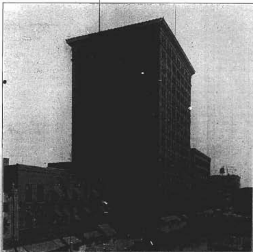
Sixteenth and Harney Streets—City National Bank Building.
