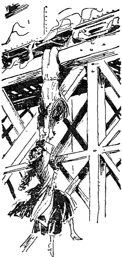
Suspended Over the Side of the Structure.
